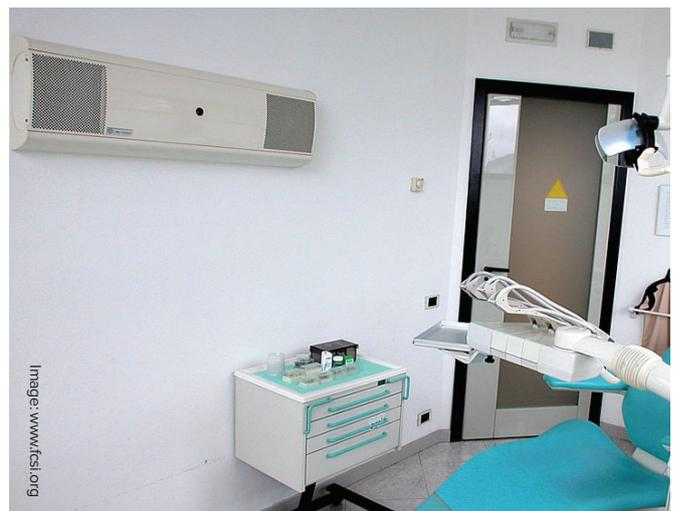
These units work by using a fan unit to draw room air into the unit. The air is passed through HEPA filters and then passed through a chamber containing intense UV lamps with reflectors and catalysts. These units can destroy most of the microorganisms that pass through them, but there is no guarantee that all room air will actually go through them. The units are typically supplied by a 230V power supply.
