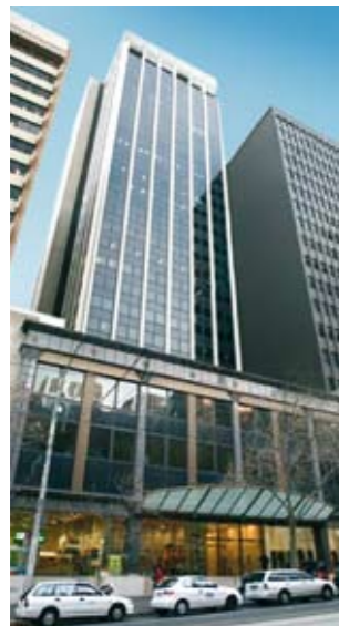
The virtually airtight facade at 500 Collins Street, Melbourne.
