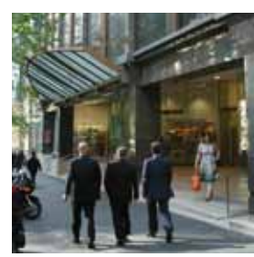
500 Collins Street, Melbourne The unique challenges of a chilled beam technology retrofit.
