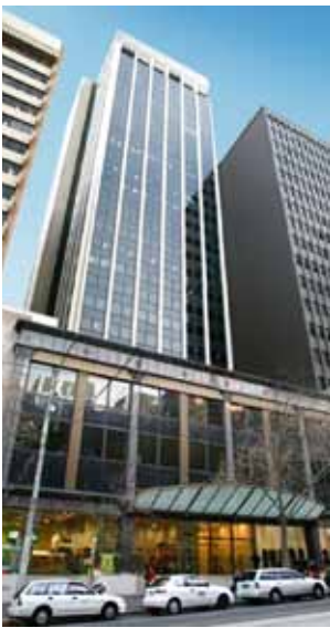
The virtually airtight facade at 500 Collins Street, Melbourne.
